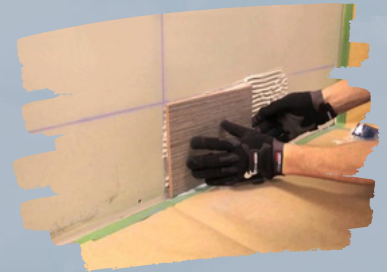
FLOOR & WALL TILING WORKS
